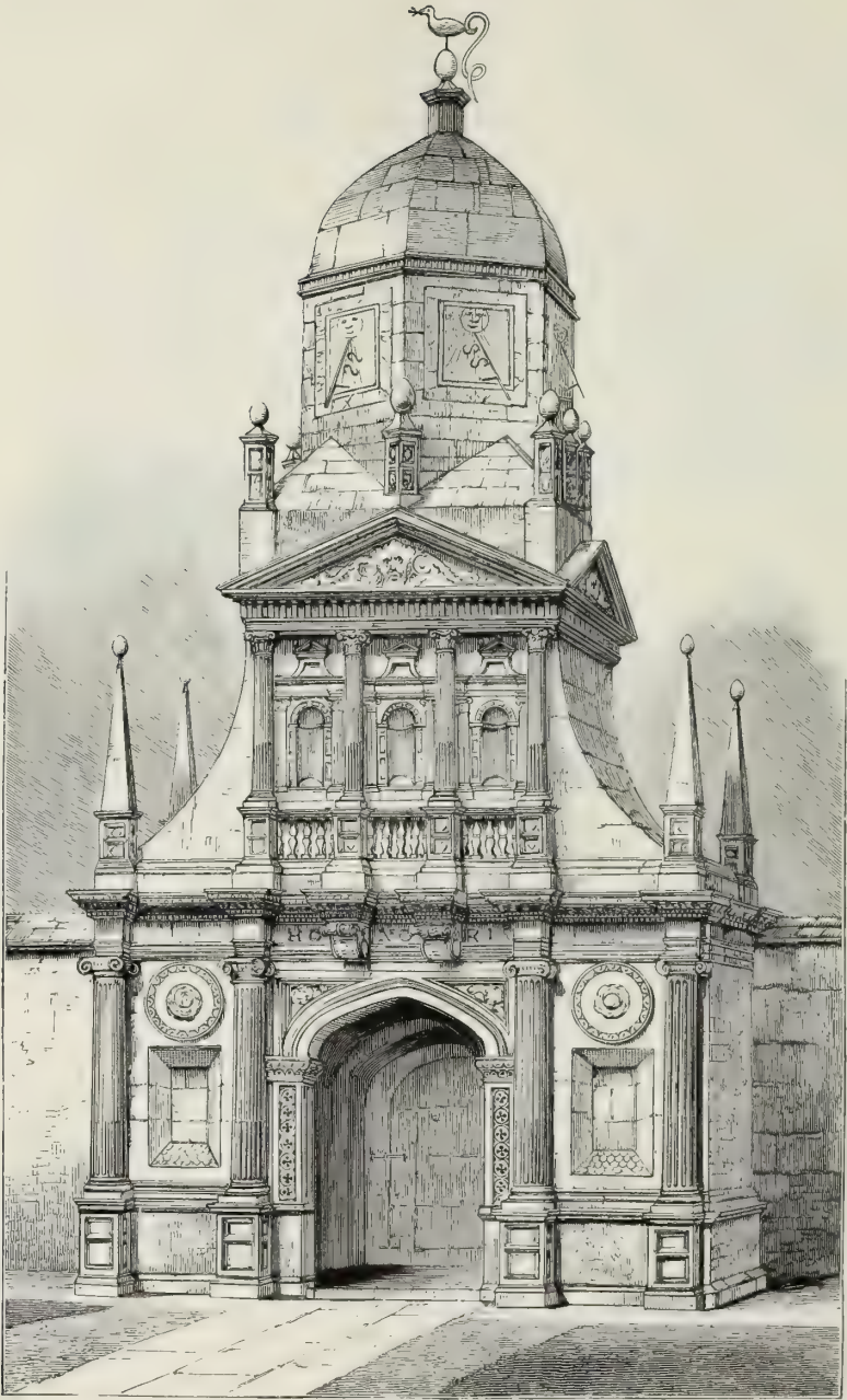
Fig. 9. Restoration of the Gate of Honour, Caius College, as seen from Caius Court.
